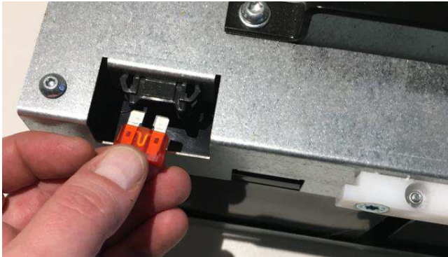
Fig. 12 | Insertion of electrical fuses
