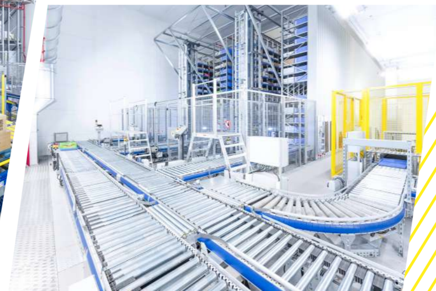
The warehouse and functional areas are directly linked to one another using a pallet and tray conveying system on three levels.
