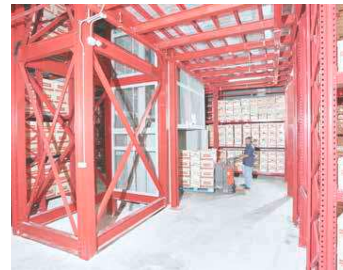
Goods lifting hoist for economic and more efficient cargo transfer between floors
