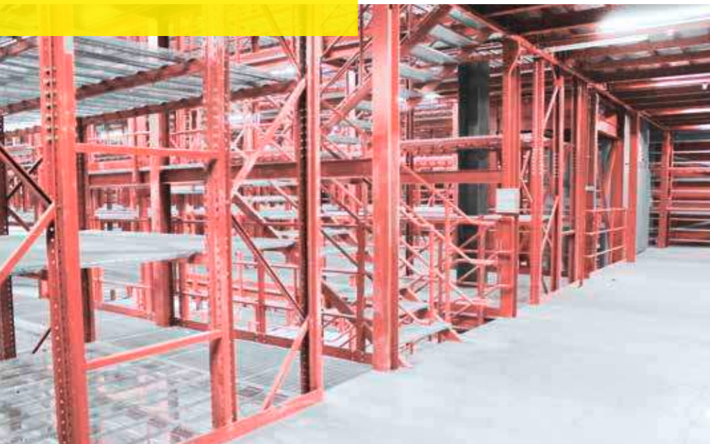
Structurally designed for maximum safety and ventilation on all levels
